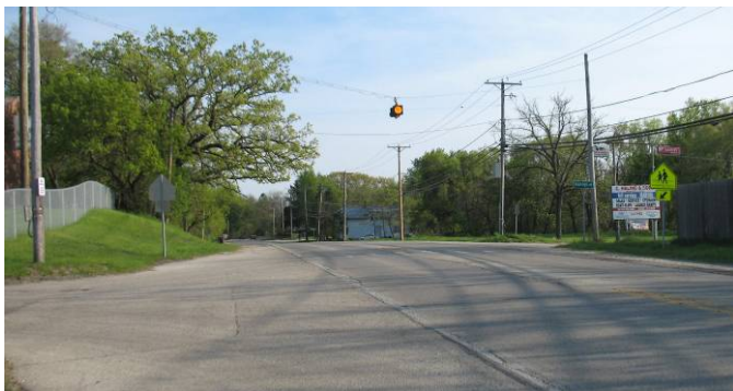
Flashing Yellow Light (coming from the East)
